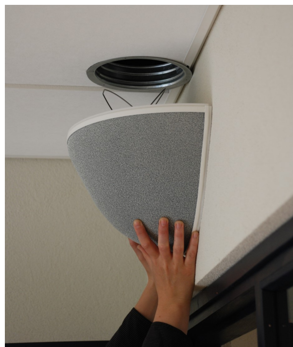
Image 2: Easy mounting with spring connection
